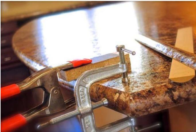
(**Fabrication Tips:** *Use a laminate faced wood block and 3" pinch clamp to maintain correct height of molding to the laminate countertop edge-see photo at left*).
